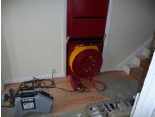
Door pressure unit to create pressure differentials
