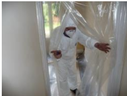
Typical controls to aid drying and prevent the spread of contamination
