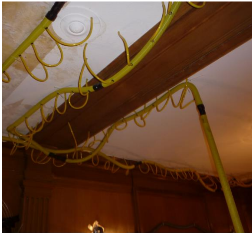
Vapour phase oxidising agent introduced into air and cavities
