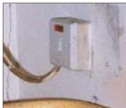
Switch to immersion heater
