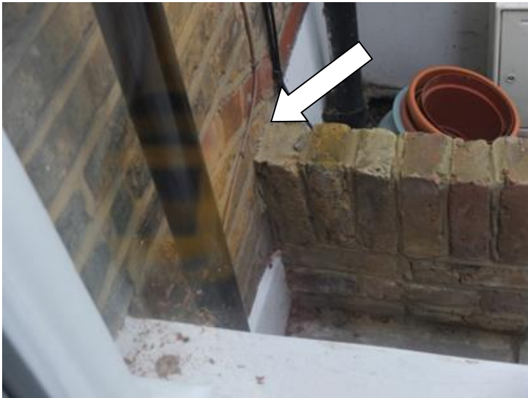
Simple construction defect where party brick wall has bridged DPC and capillary action caused internal damp & mould growth
