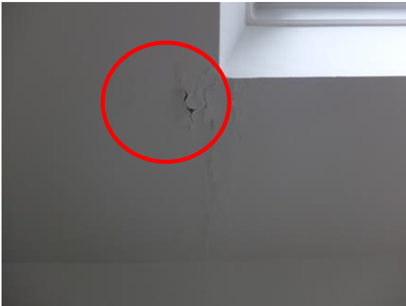
A minor leak from poor window installation led to major mould growth in ceiling cavity which leached out through downlighters etc
