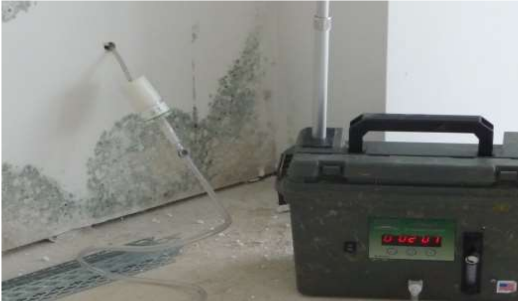
42 New construction where builders removed surface mould and stated only redecoration was necessary
