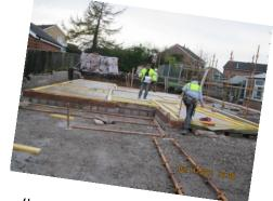
much lighter than a traditional block and brick-built house (by a factor of up to 75%), there is much less chance of movement of the structure in the decades ahead as the foundations are under much less stress.
