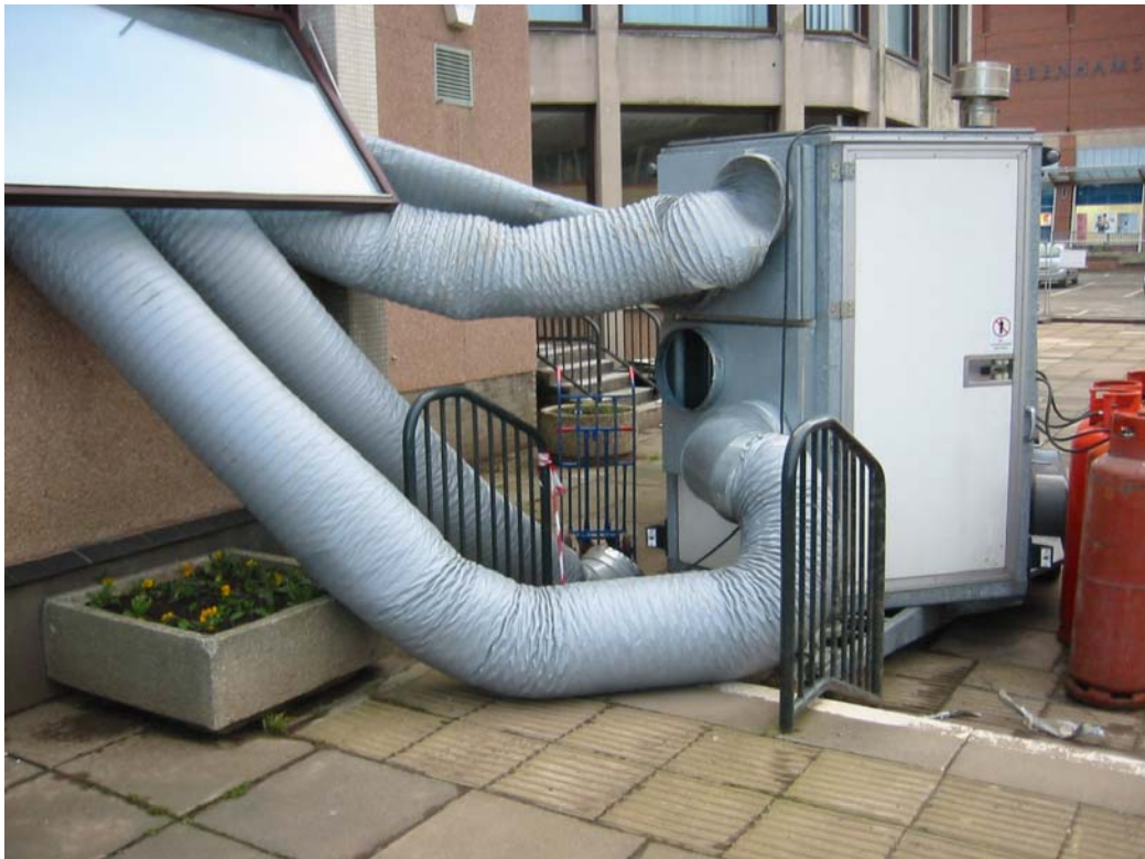
This photo shows a trailer mounted system poorly installed with a collapsed hose, top, and disconnected hose bottom. The windows are not sealed either
