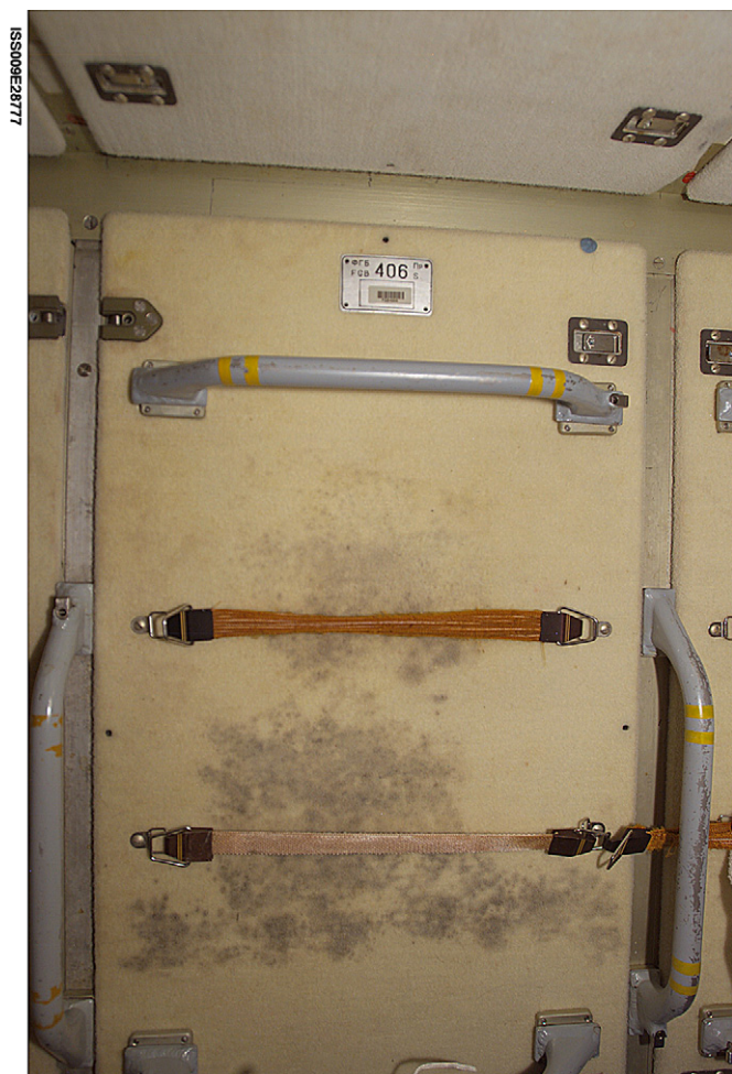
Fig. 1. Mold-stained panels in the ISS hygiene area resulting from mold growth following contact with wet towels. Approximate area affected is 2 m 2 .
