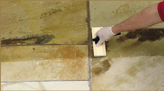
R R Sandstone Seal is applied in one or more light coats by Sponge Applicator, short fibre roller or soft brush to the clean dry surface until a uniform matt or low sheen finish is obtained. Previous coats must be tack free before the next is applied.
